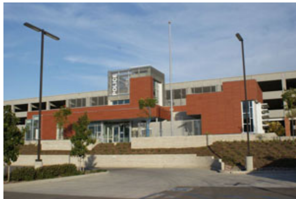
Designers of the Miramar College campus police station are aiming for LEED Platinum certification
