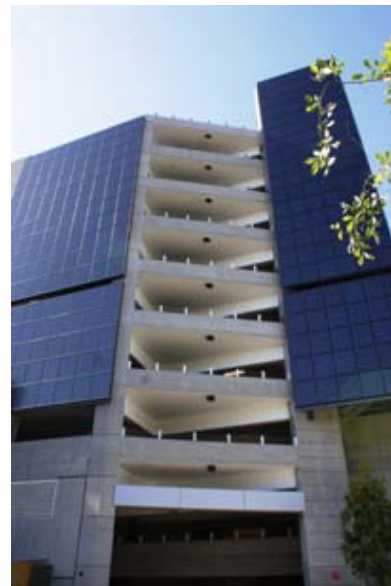
The vertical array on the south facade of the City College Career Technology Center parking structure is the largest of its kind in the country.
